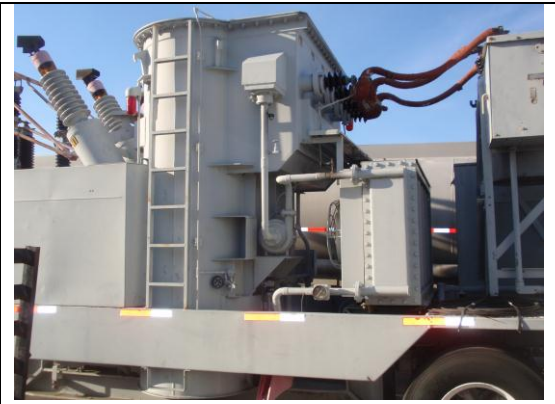
7.5 MVA 67 x 13.8 – 2.52/4.36Y x 5.04/8.72Y x 7.56/13.09Y GE
