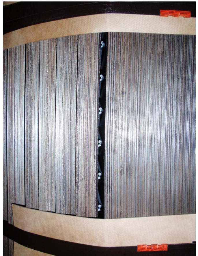
Installation of 1/4" Oil Ducts
