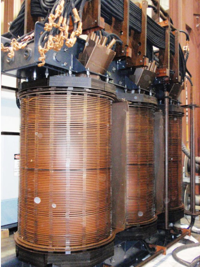
Leads coming out of just the top of the coils
